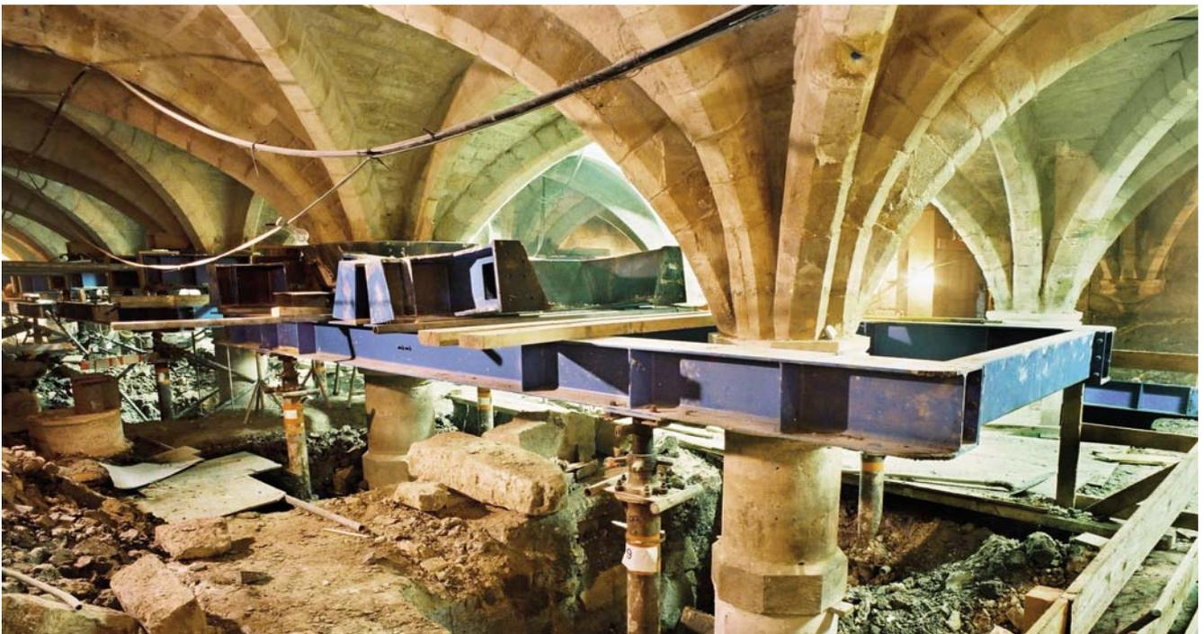
*Pillars underpinned by a metal collar resting on micropiles*
